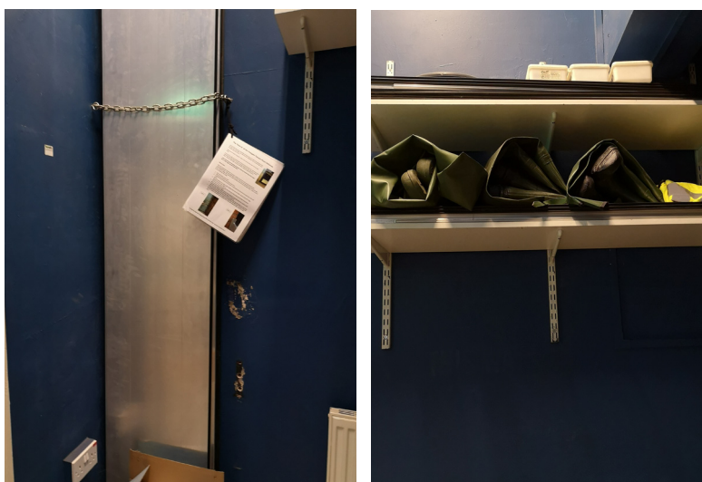
Photo 47: Flood gate boards with instructions Photo 48: Kits for flood
