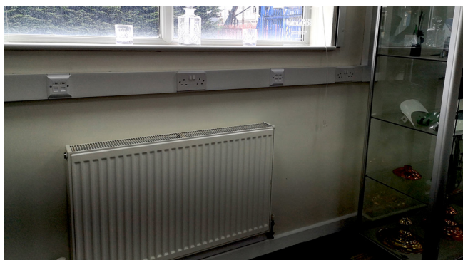
Photo 5: Raised electrical points
