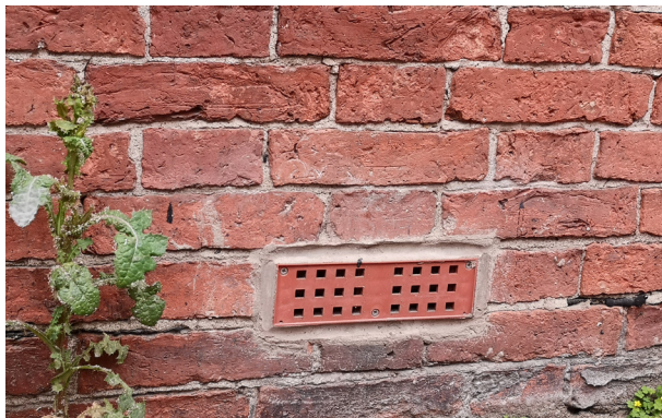
Photo 49: Air vent on the wall
