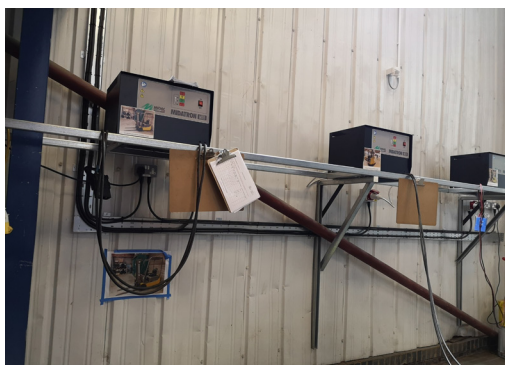
Photo 7: Forklift chargers on raised shelf
