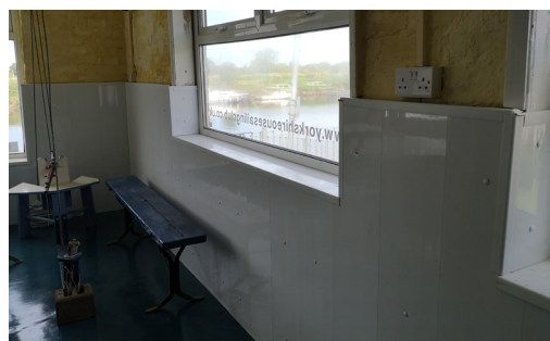
Photo 29: Raised electricity sockets
