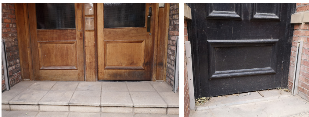
Photo 45/46: Flood gates at the external doors
